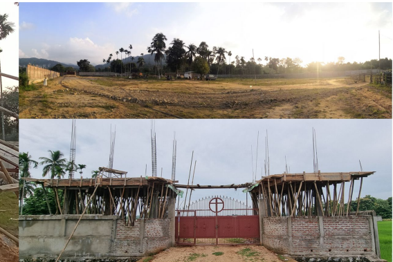
12. MAIN ENTRANCE GATE
